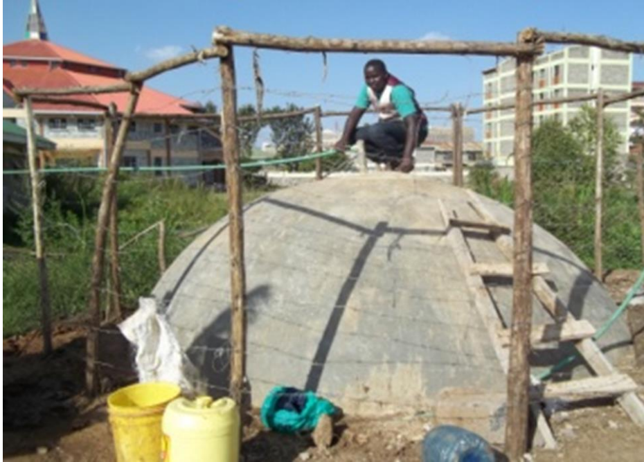
Biogas Digester at the St. Francis Street Boys Rehabilitation Center, boys here learn by doing. From the streets of Nairobi, they are becoming farmers.
